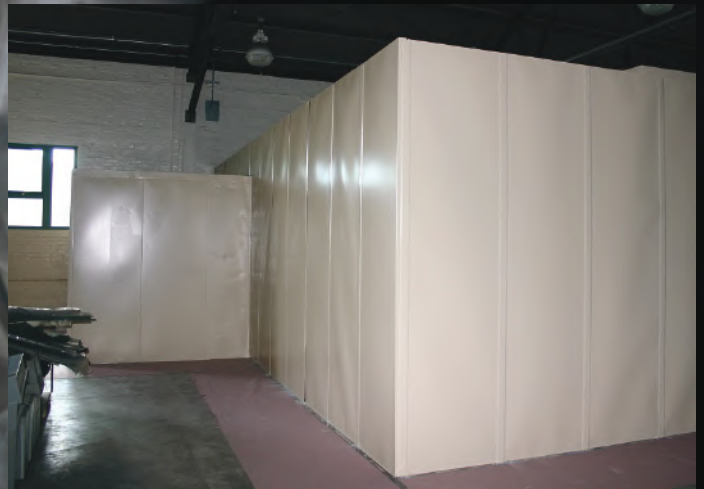
FINISHED LIGHTWEIGHT™ VAULT WITH LIMITED ACCESS
