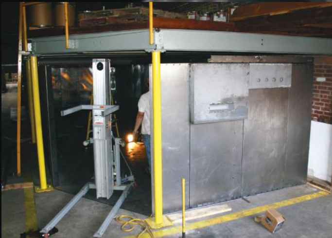
LIGHTWEIGHT™ VAULT INSTALLED UNDER A PRE-EXISTING MEZZANINE
